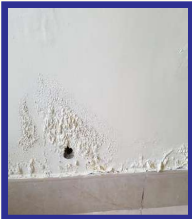
WALL DAMPNESS TREATMENT
