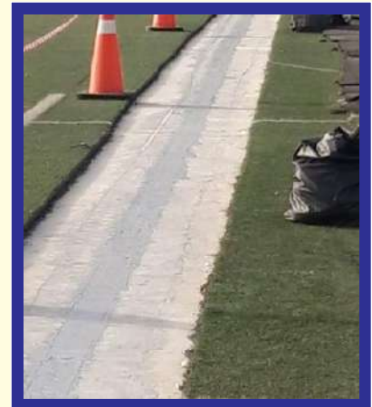
EXPANSION JOINT WATERPROOFING
